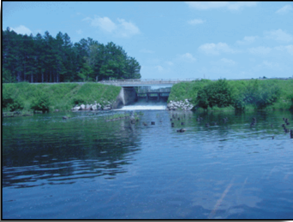
Rest Lake Dam
